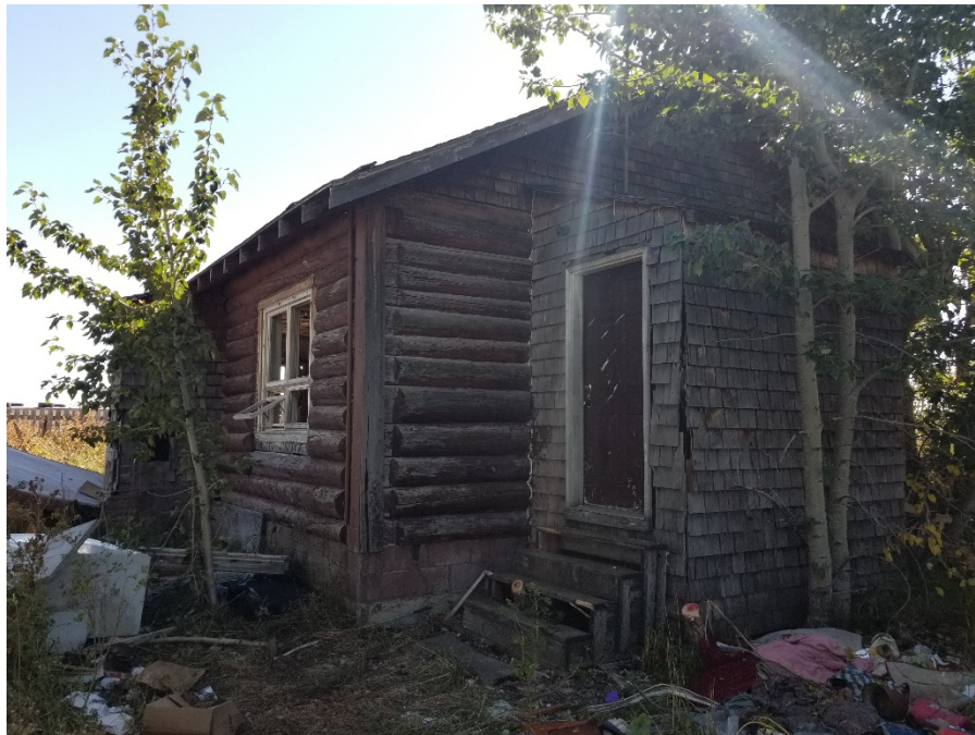
Photo 4. Project close-out photo Rutherford House looking northeast.
