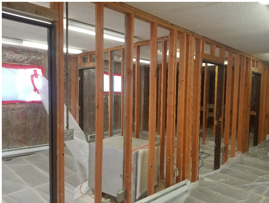
Photo 12. Final clearance project photo taken inside the Community Center looking southwest.
