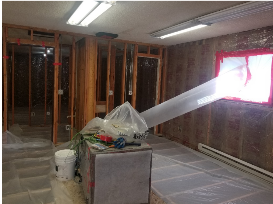
Photo 11. Final clearance project photo taken inside the Community Center looking northwest.
