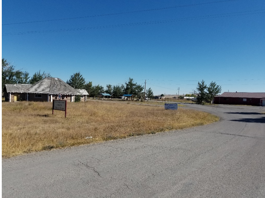
Photo 1. Entrance to Heart Butte Government Square. This photo shows the proximity of the Round Hall and Community Center.
