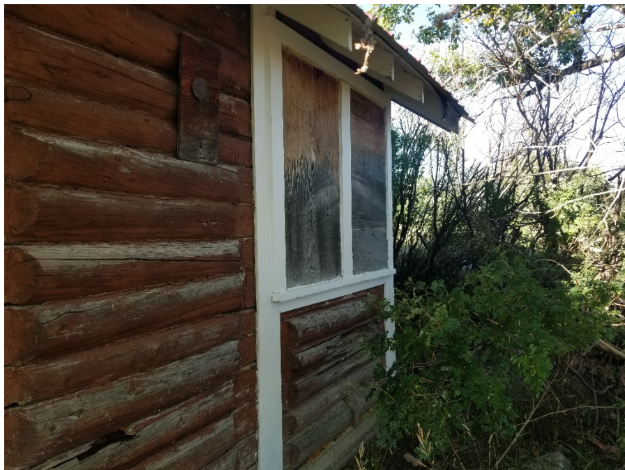
Photo 10. Project close-out photo for lead abatement and repainting of exterior window trim on the Comes at Night House.
