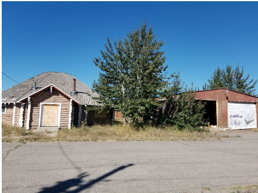
Photo 2. Project close-out photo looking southwest at the Round Hall and Fire Garage.
